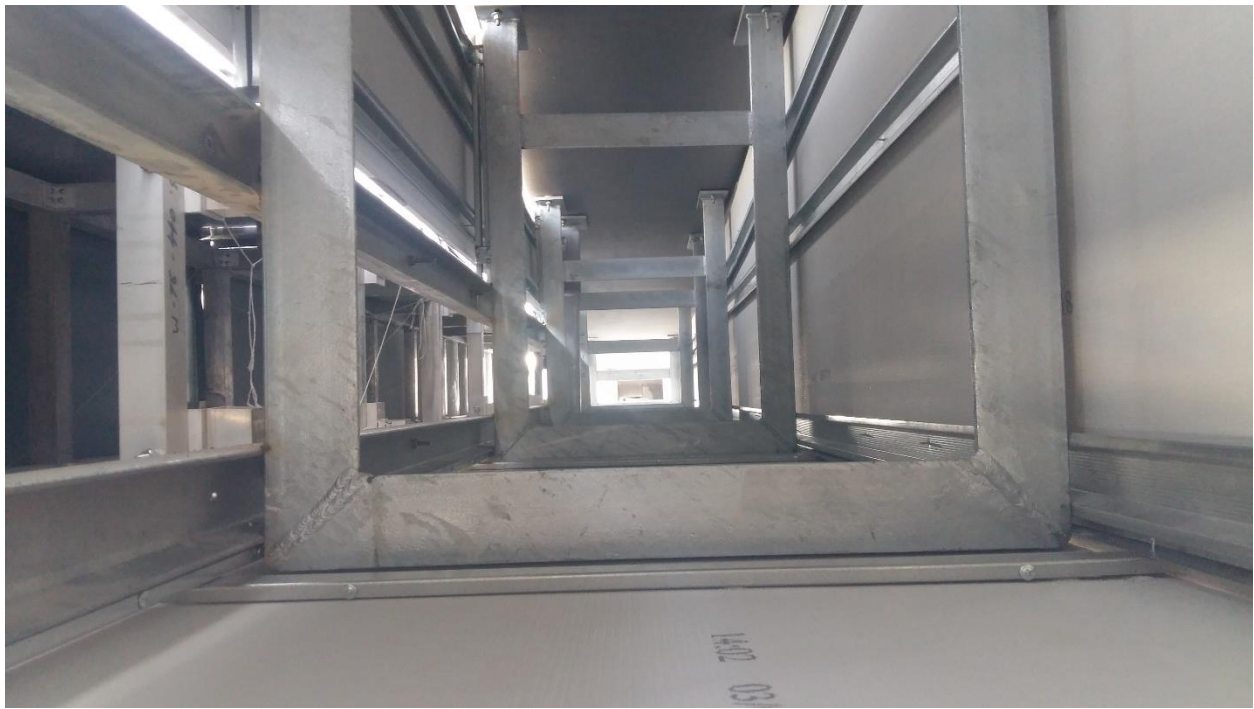
SECONDARY STEEL WITH GYPSUM CLADDING FOR FAÇADE
