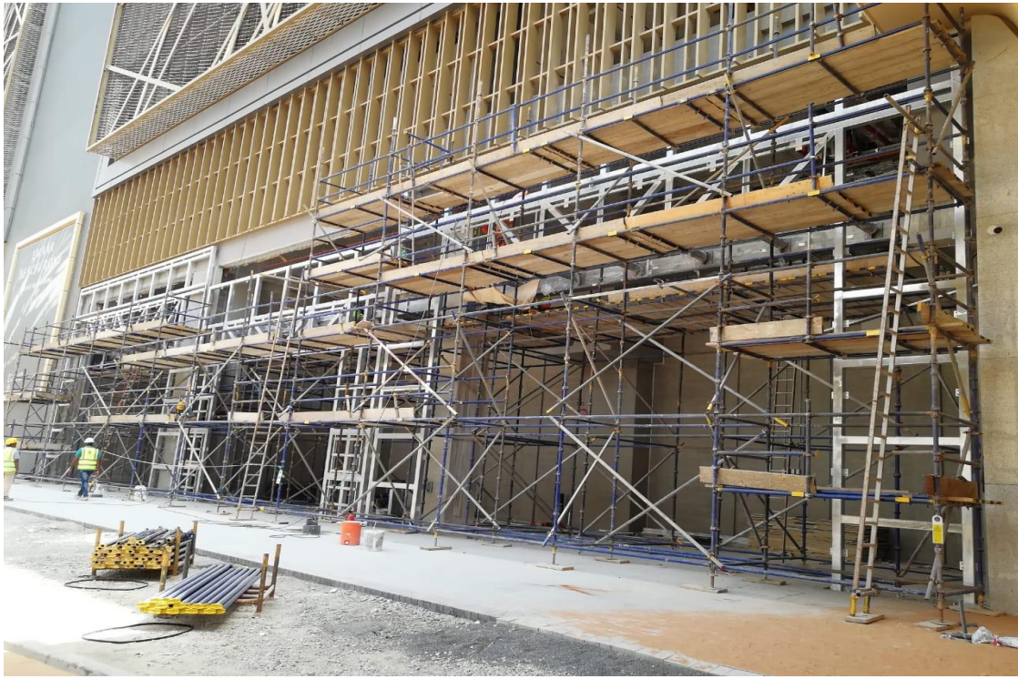
SECONDARY STEEL FOR CLADDING
