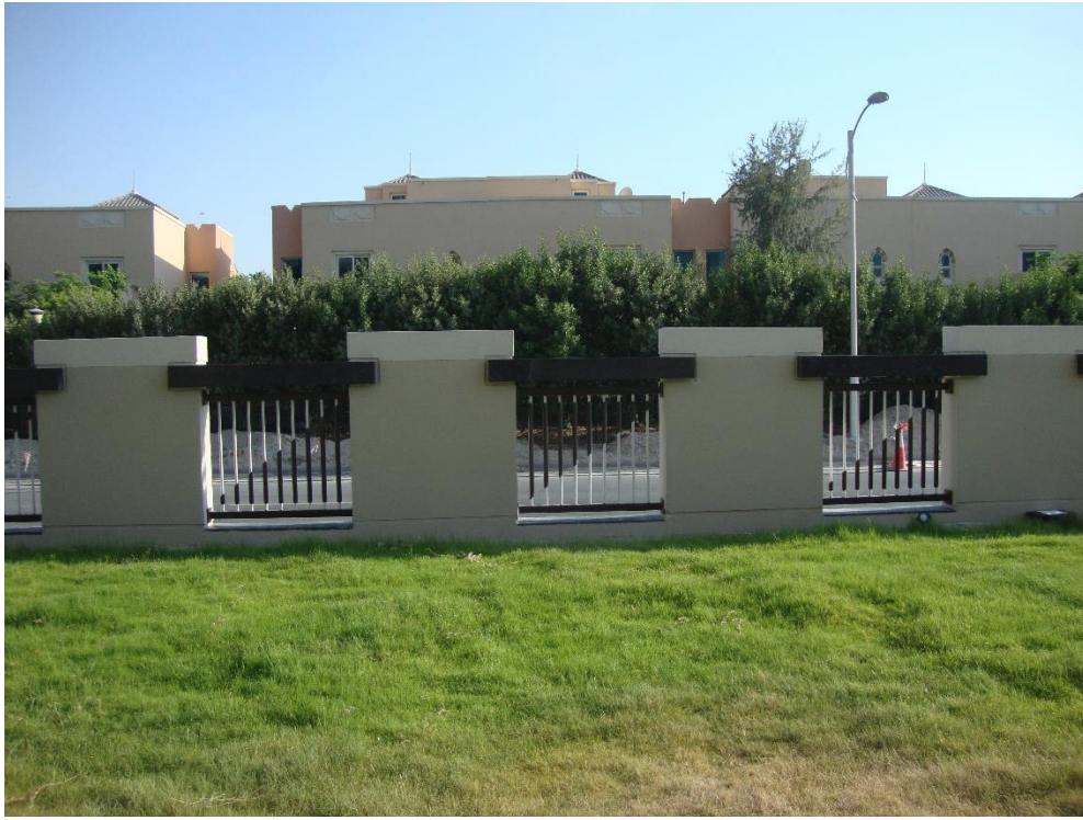
EXTERNAL BOUNDARY FENCE
