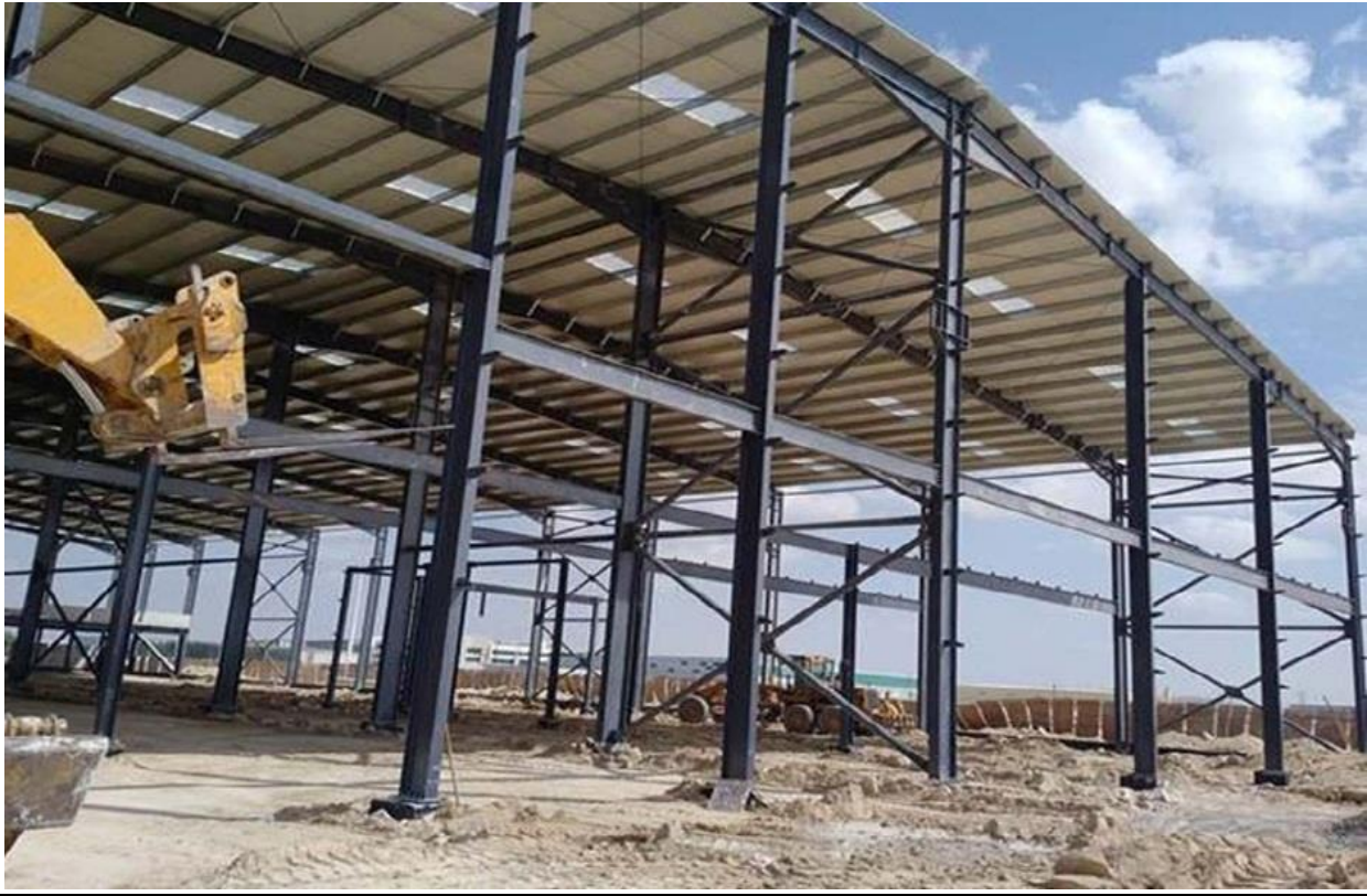
INDUSTRIAL SHED (TOTAL STEEL – 700 TONNES)
