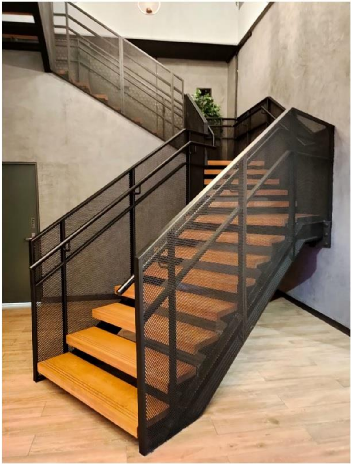
ARCHITECTURAL METAL STAIRCASE
