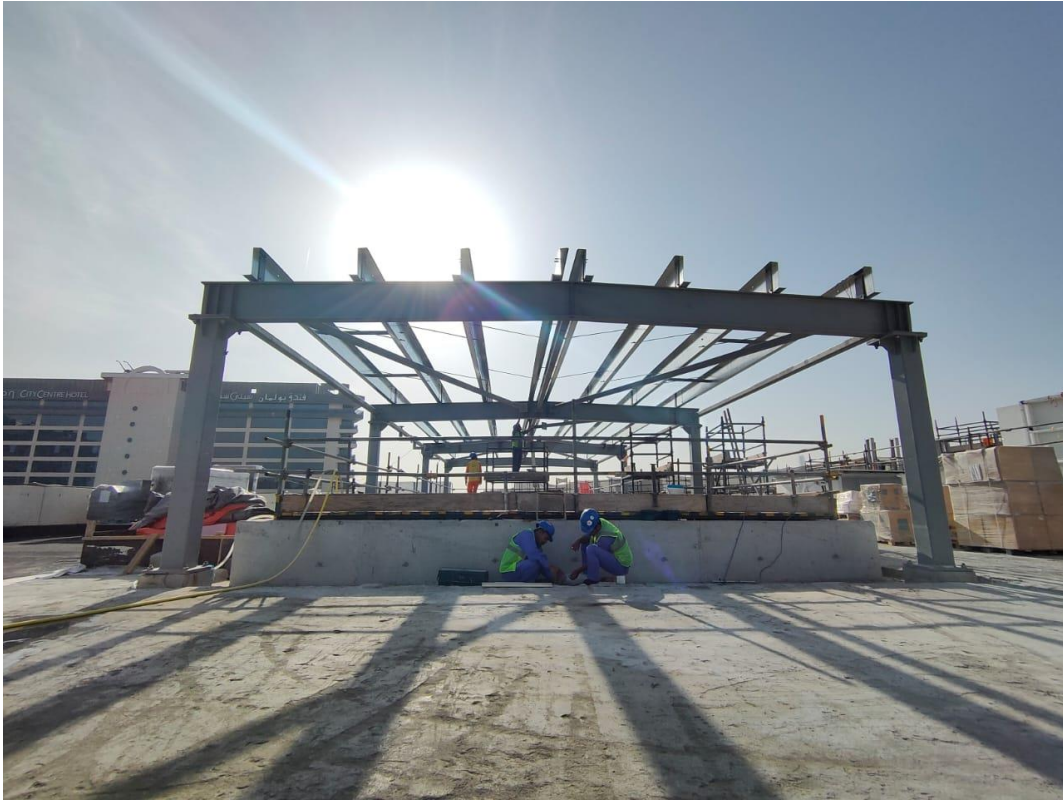
STEEL STRUCTURE FOR SKYLIGHT ON ROOF
