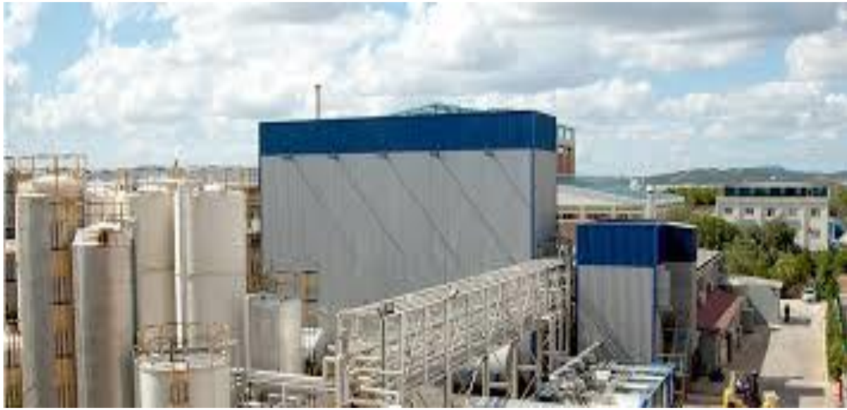
KMT POLYMERS FZC – STORAGE TANKS & PROCESS EQUIPMENTS
