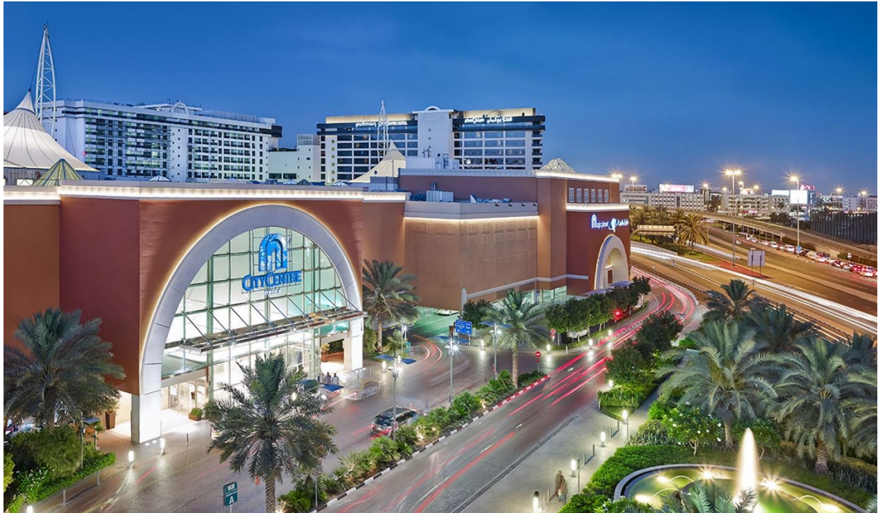
DEIRA CITY CENTRE REDEVELOPMENT (OWNER – MAJID AL FUTTAIM, MAIN CONTRACTOR – DUTCOCONSTRUCTION)
